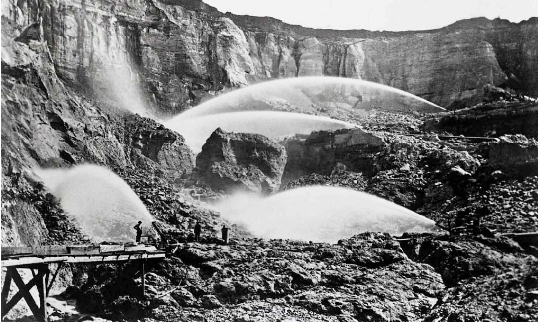
Figure 191. Hydraulic mining at Malakoff Diggins. Water cannons washed the gold-bearing soil and gravel from the hillside. (Photo courtesy California State Parks Photographic Archives.)
