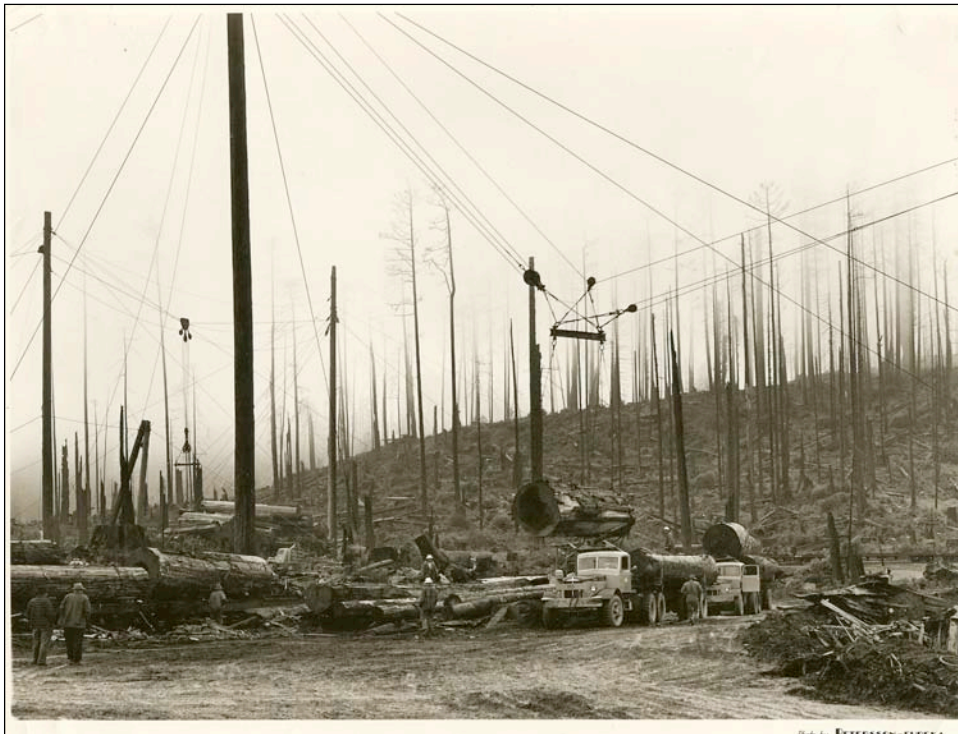
Figure 200. Sky-line cabling moves logs to landings with the whole log suspended on cables. Both high-lead and sky-line cabling systems require the removal of trees and brush along the route to prevent the logs and cables from getting tangled in the intervening trees. Compare this picture with Figure 212, page 142. (Photo courtesy Clarke Museum Collection.)
