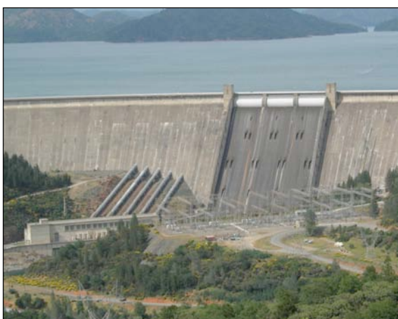
Figure 220. Shasta dam and electric power generating facility.
