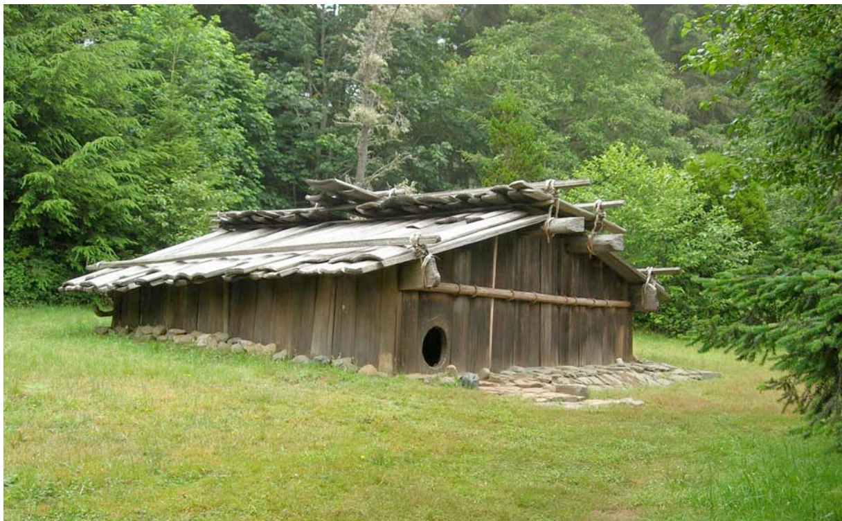
Figure 182. This replica of a Yurok redwood plank house can be seen at Patrick's Point State Park, north of Arcata. Note the small entrance opening, which helps conserve heat and makes the dwelling more secure. Since the house surrounds a pit, the walls didn't need to be very tall.
