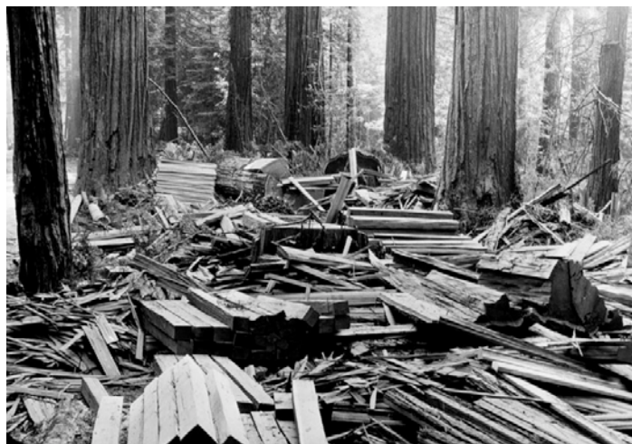
Figure 186. Coast redwood made excellent railroad ties. The old-growth wood used in the 1800s and early 1900s was relatively knot-free, so it split easily. The tannins in the wood made it rot- and insect-resistant. Note the tremendous amount of wasted wood. (Library of Congress photograph.)
