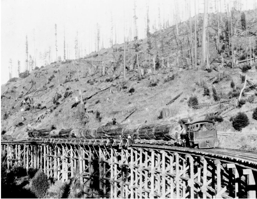
Figure 201. The rugged terrain of northern California required the building of some impressive railroad trestles. Note the nearly clear-cut hillside, and also that young trees have started to grow. For scale, see the man standing on a log near the middle of the train. (Photo courtesy of Humboldt Redwood Company, formerly Pacific Lumber Company.)
