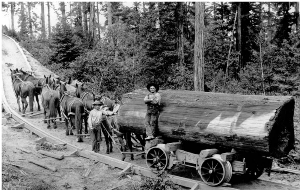
Figure 202. Temporary horse- or mule-drawn “railroad” with wooden tracks. Sometimes logs were used for tracks instead of boards. Note the wide wheels on the cart. (Photo courtesy of the California Redwood Association.)
