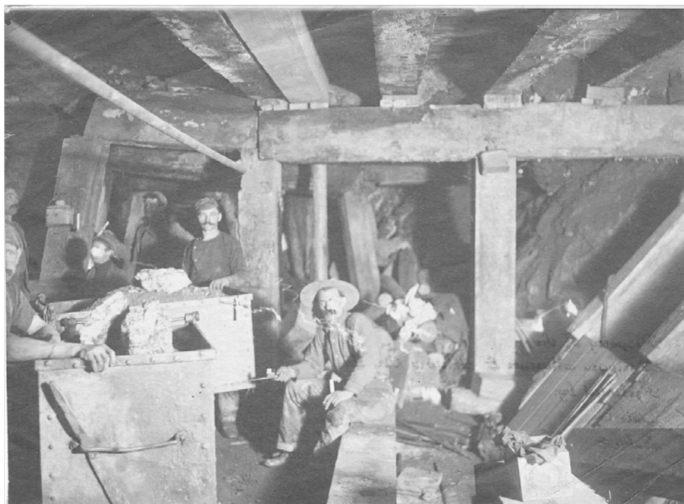
Figure 190. Mine tunnel at the Princeton Mine, near Mariposa, CA. Mines needed timber for shoring up the walls and ceilings as well as for buildings and fuel for stamp mills and other machinery. (Photo courtesy Mariposa Museum and Historical Center Incorporated.)
