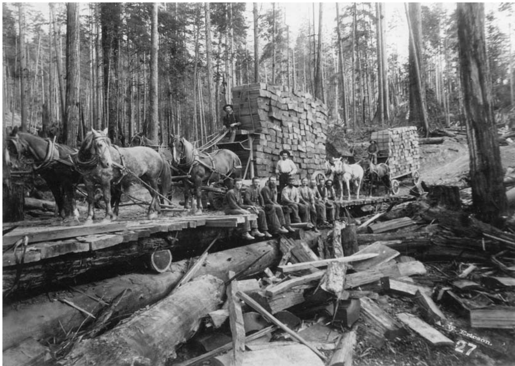
Figure 204. Shingles and boards were needed for building houses. Redwood’s resistance to rot made it ideal for shingles, grape stakes and railroad ties. Here “split product,” probably shingle wood, is moved by horse-drawn cart to a shingle mill, port or railroad loading area. (Photo courtesy Clarke Museum.)
