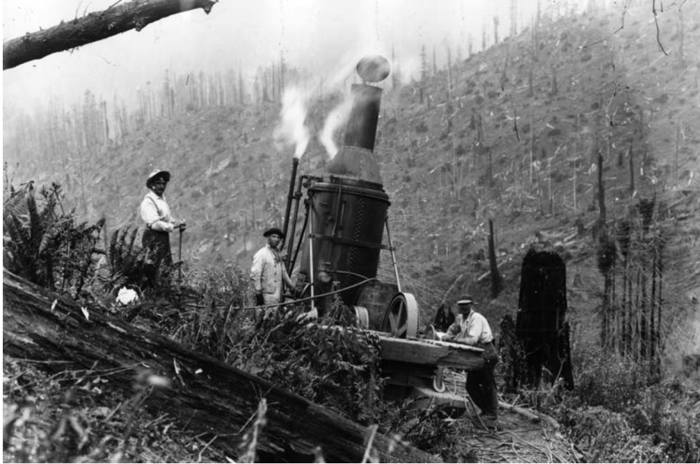
Figure 199. The Dolbeer Donkey engine, named for its inventor, John Dolbeer, who was a partner in the Dolbeer and Carson Lumber Company of Eureka, made it easier and faster to move logs to a landing. It also was hard on the forest plants and soil. (Photo courtesy Humboldt State Library Humboldt Room Collection.)
